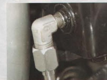
The flare nuts are tightened down and the job is finished.
